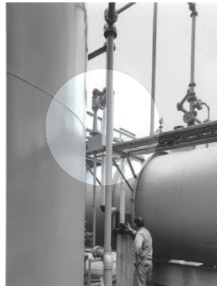
Stock Fig. 7014 scrubber system, used to remove HCL fumes during tank venting, illustrates the benefits of a compact lightweight system.
